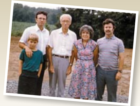
Marvin and Rosella McColpin (center) visited the site of 3ABN's first building as the foundation was being dug. Danny (right) and Kenny Shelton (left) showed them around, with Kenny's son, Jeremy.
