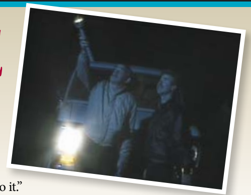
Clarence Larson and Danny Shelton were surprised to find three-phase power near the building site.
